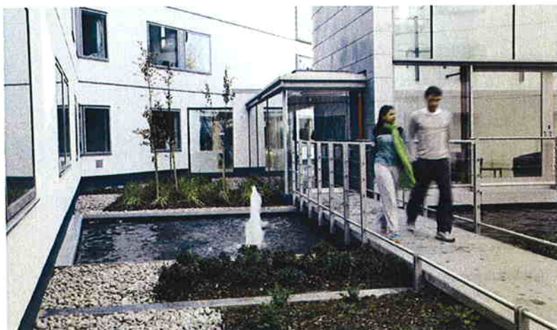
Right A six-storey wing juts out in front of the main entrance and presents a blank zinc-faced wall to the noisy railway viaduct
