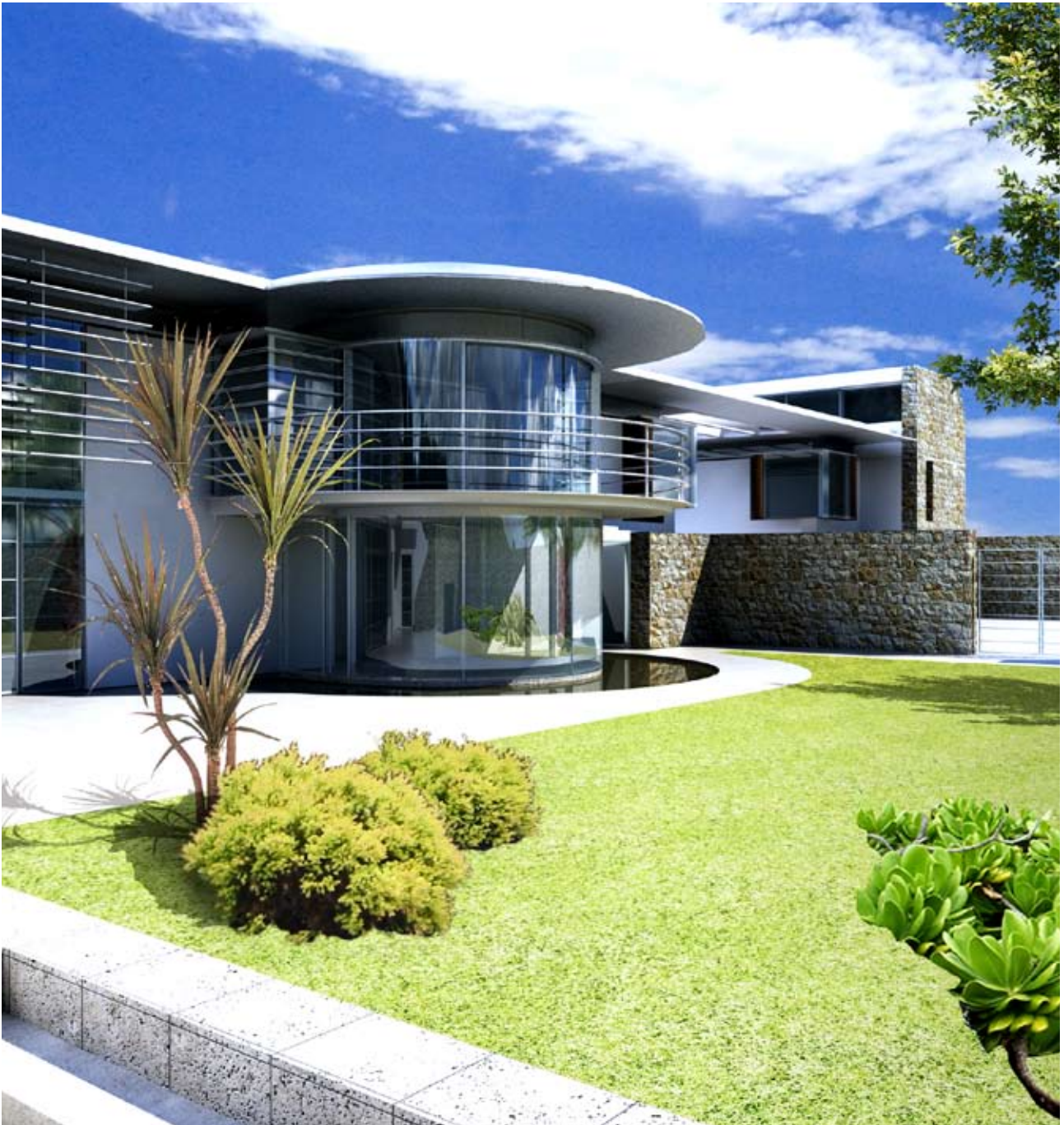
View of south elevation from sunlit garden
