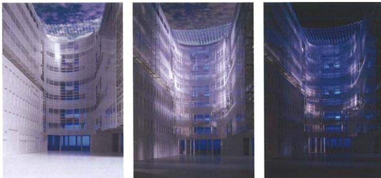
A model of the proposed redevelopment of Broadcasting House illustrating the translucency of the façade during the day and its transparency at night.
